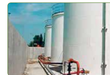
Fluid tight structures
