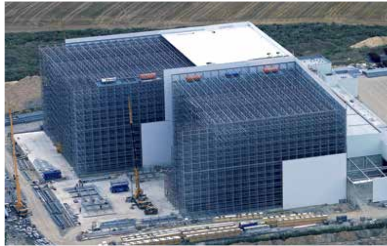
Figure 10: A typical clad rack system
