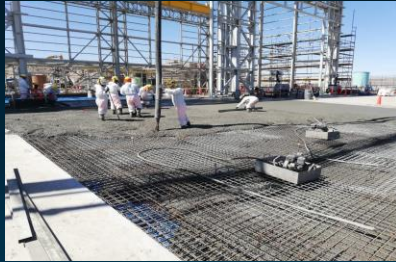
Heavy, labor-intensive traditional reinforcement
