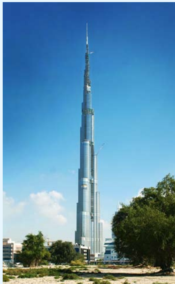
At a height of 818 meters and with 160 habitable floors, Burj Dubai is the highest skyscraper in the world to date.
