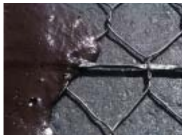
Road reinforcement – Meshtrack Reduced deformation in the asphalt overlay.
