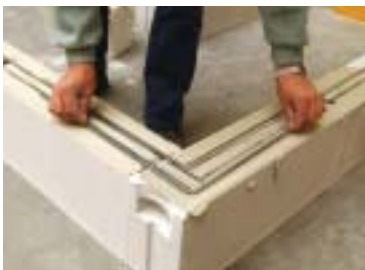
Wall reinforcement for masonry – Murfor Prevents cracking and increases the resistance of the wall.
