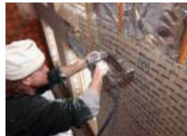
Welded lath for plastering walls and ceiling - Stucanet Light, strong and easy to shape.
