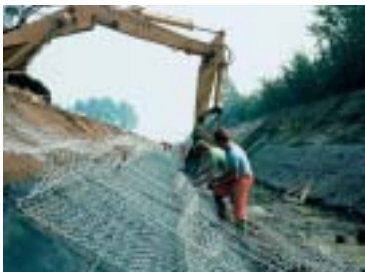
Rock protection Guaranteed strength and rigidity by use of profiled wires.
