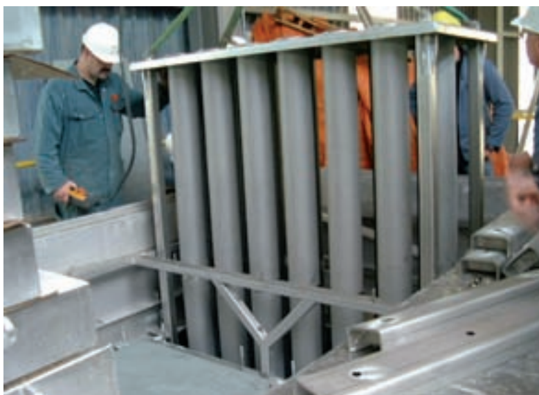
Installation of filter elements
