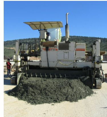
Slip form paver machine
