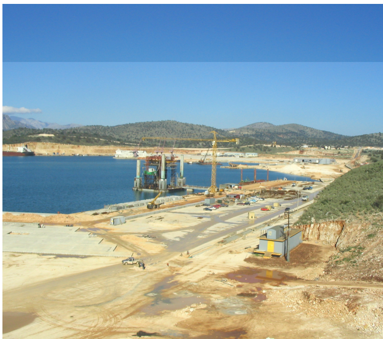
View of the harbour
