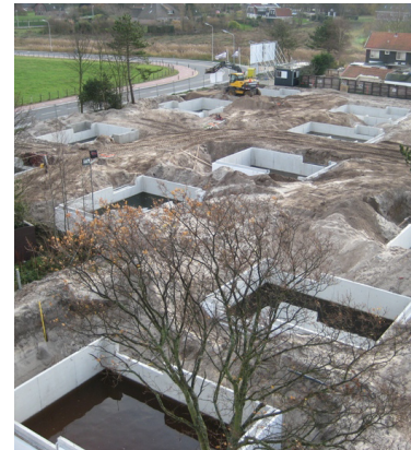
overview of job-site
