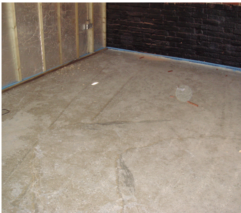
Finished Dramix RC-80/50-BN floor ready for tile fixing
