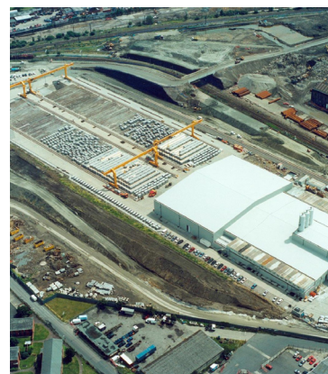
Temporary Precast Factory at Stratford over 200000 segments produced
