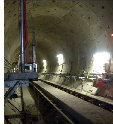
South bound bore nearing completion
