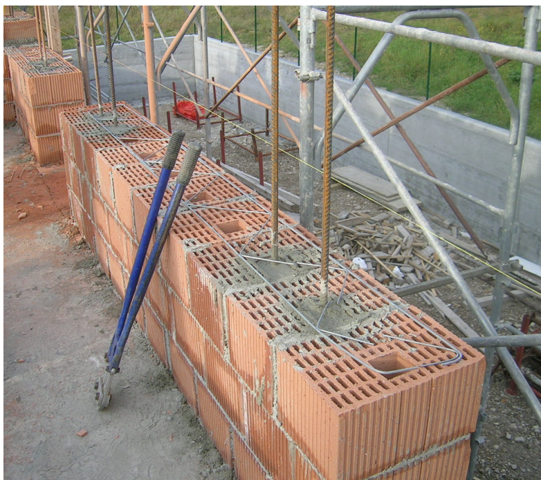
Reinforced masonry with Murfor
