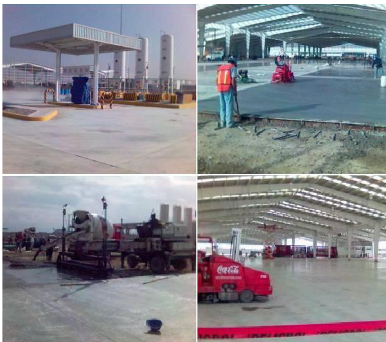
Gas filling station - Vibrating + laser screed - Warehouse
