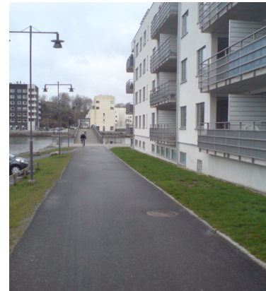
Picture showing typical balcony
