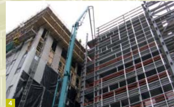
4 No problem to pump, even 200 meters high
