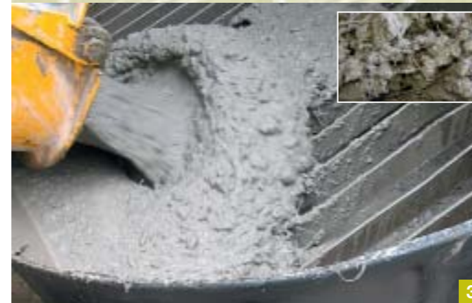
3 A homogeneously mixed Dramix® concrete is delivered on the jobsite
