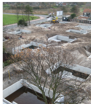
overview of job-site
