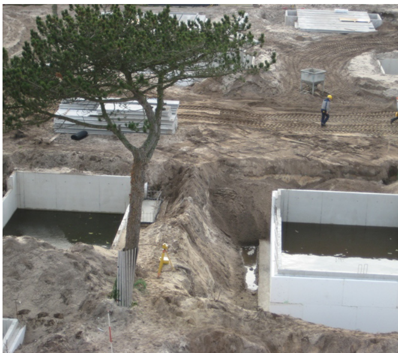
concrete delivered by BEMA Alkmaar (60 % Mebin- Heidelberg group)
