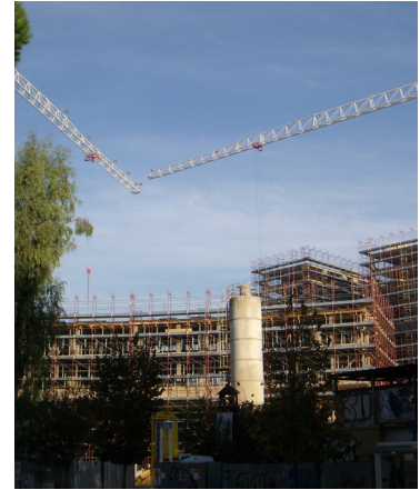
n.2 buildings under construction
