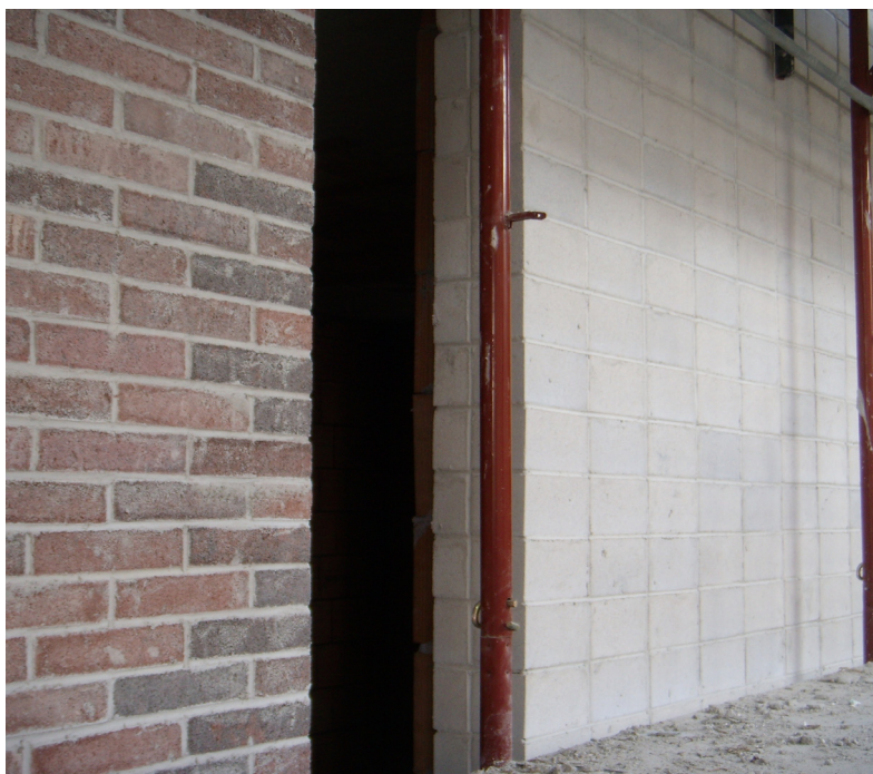
Standard and unbonded masonry
