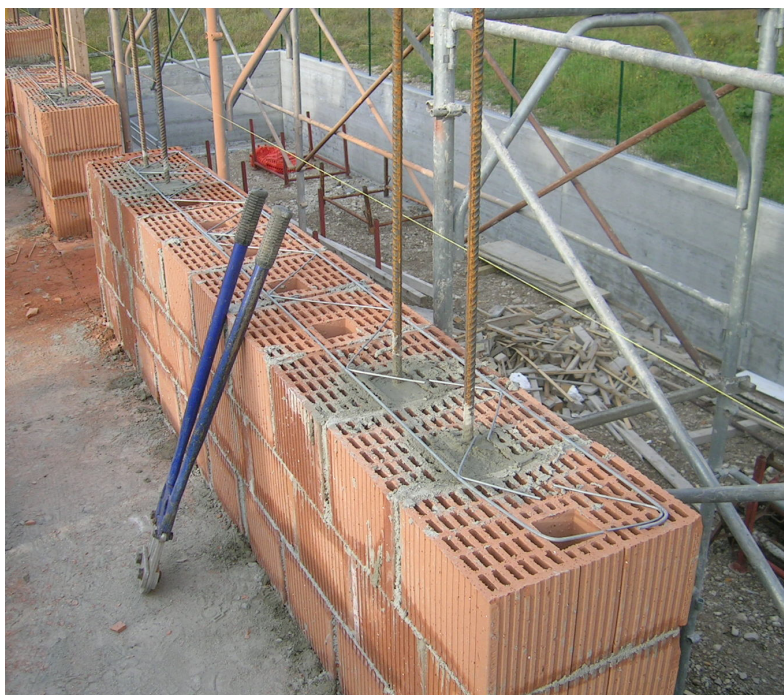
Reinforced masonry with Murfor
