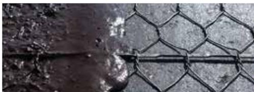
Mesh Track® is a steel-based structural asphalt reinforcement solution that has been around for more than 30 years. Whereas roads with a typical top layer need renovation every 5 year, Mesh Track® delays this need by 20 years or more. Working with Mesh Track® also speeds up construction, as the underlying pavement structure does not need to be exposed. As a result, road renovation with Mesh Track® is not only more durable, but significantly more cost-effective than building a new road.
