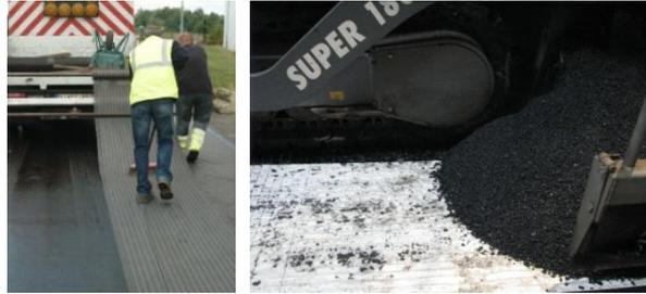
**Fig. 1** Installation process of the new flexible steel-based anti-cracking interlayer
