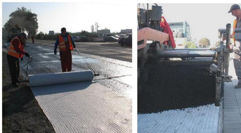
Figure 2: Installation process of the new steel-based anti-cracking interlayer with non-woven on a ground concrete surface
