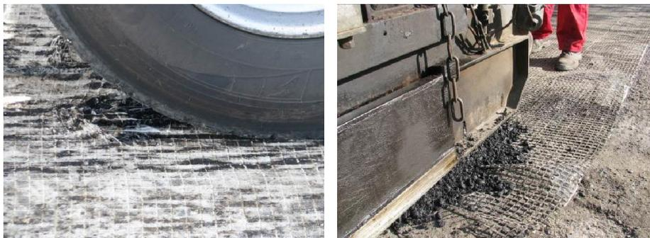
Figure1: Left: Due to tackiness, the product is damaged by traffic. Right: A wrinkle in a geogrid inducing a discontinuity in the asphalt.
