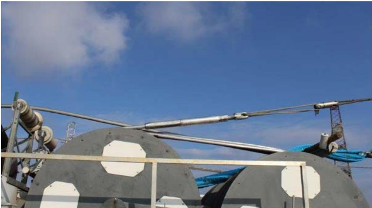
During sagging, the conductor was supported by 4 wedge type grips, disposed in a double tandem configuration as show in picture 4.
