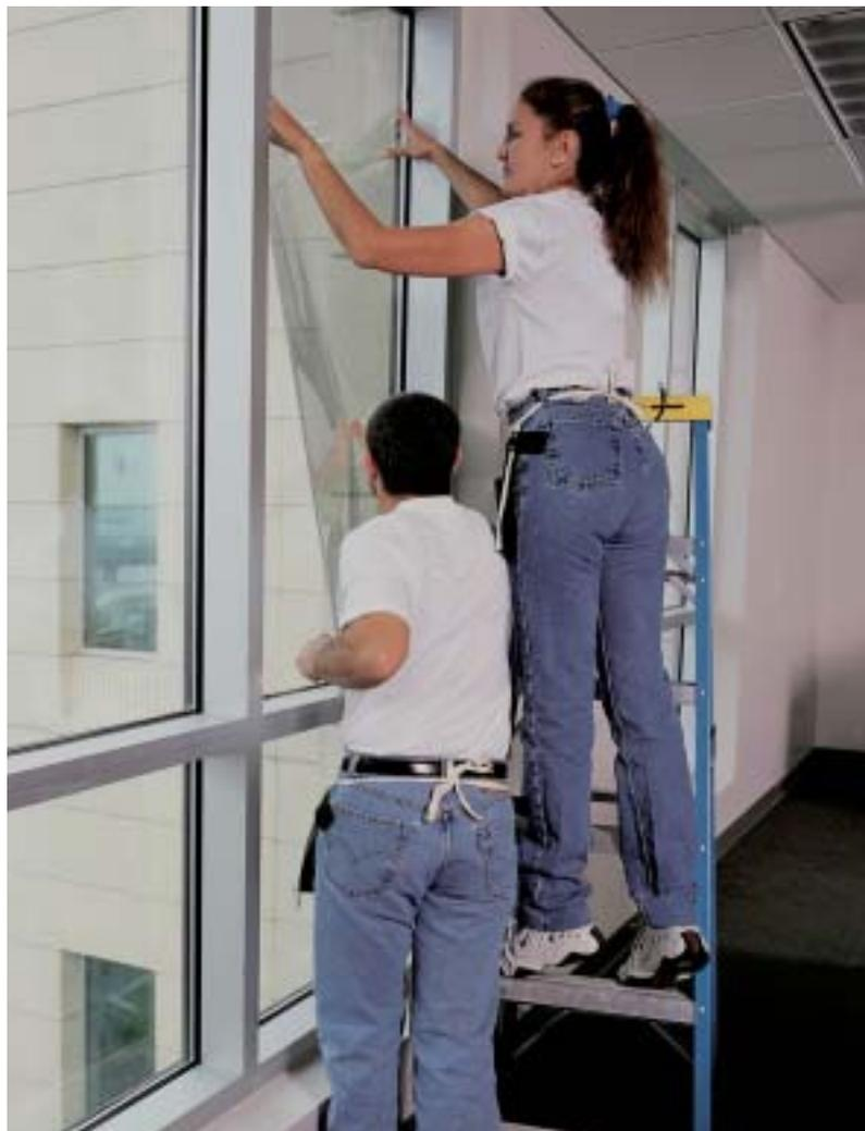
Specialized installers applying window film to keep out the sun's heat and ultraviolet radiation and provide protection in the event of breakage.
