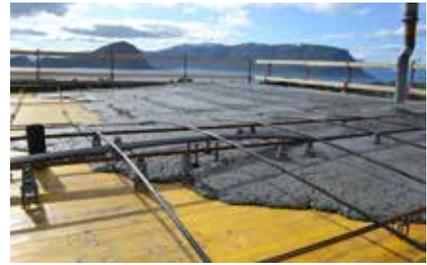
*Mix of Dramix® and post-tensioning replace traditional passive reinforcement in on-grade applications*
