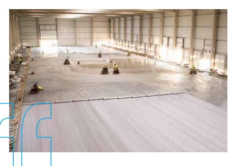
A 10,000 m² high-performance and completely seamless floor was cast for CDC Germany within just a few days. It consisted of two panels of 120 m x 42 m without any joints. The design was made possible by SigmaSlab®, a concrete reinforcement technology which combines CCL's post-tensioning systems with Dramix® steel fibers.
