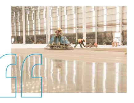
Retail giant Coppel constructed a 47,000 m², heavy-use distribution center in Texcoco, Mexico, using SigmaSlab® concrete reinforcement technology - a first for Latin America and only the second worldwide. The technology, combining Dramix® steel fibers with CCL's post-tensioning strands, produced a high-performance floor with substantial time and cost savings and eco-friendly advantages.
