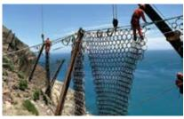
In order to improve the endurance of rock protection netting, Bezalplast® is used to protect the wire from the elements.
