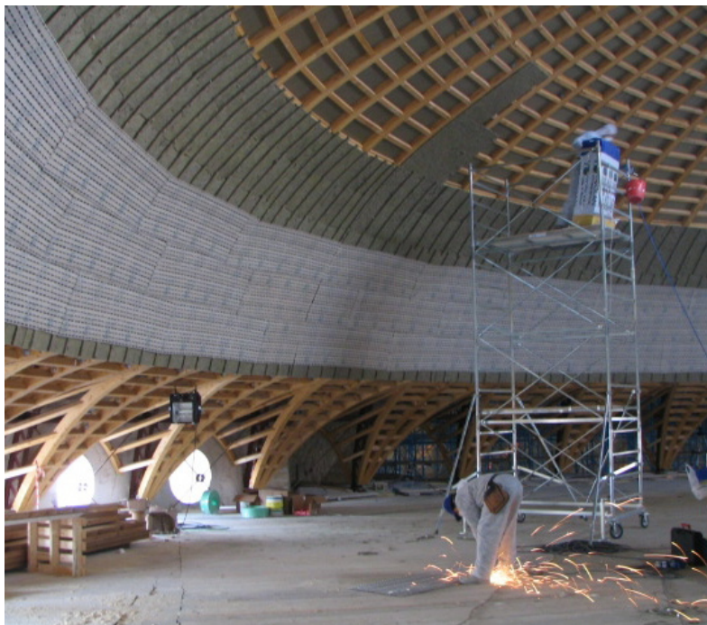
Installation of Stucanet panels
