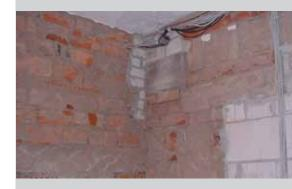
The substrate in renovation projects often consists of a mix of different building materials. Bekaert Stucanet<sup>®</sup> allows the durable renovation and plastering of this type of difficult walls.
