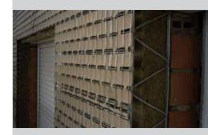
Bekaert Stucanet<sup>®</sup> as mortar support in a facade insulation system, mounted on metal Bekaert Poutrafil<sup>®</sup> profiles.
