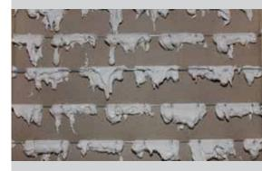
The bonding of the mortar around the steel wires ensures firm anchoring.
