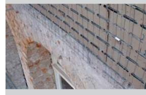
Bekaert Stucanet® applied in a facade renovation project with exterior plasterwork.
