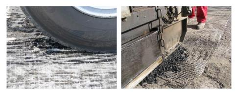
Figure1: Left: Due to tackiness, the product is damaged by traffic. Right: A wrinkle in a geogrid inducing a discontinuity in the asphalt.
