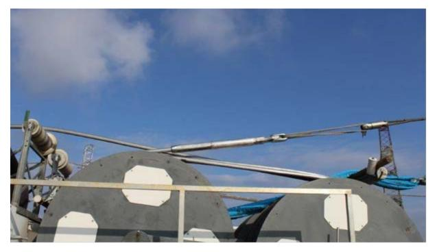
During sagging, the conductor was supported by 4 wedge type grips, disposed in a double tandem configuration as show in picture 4.
