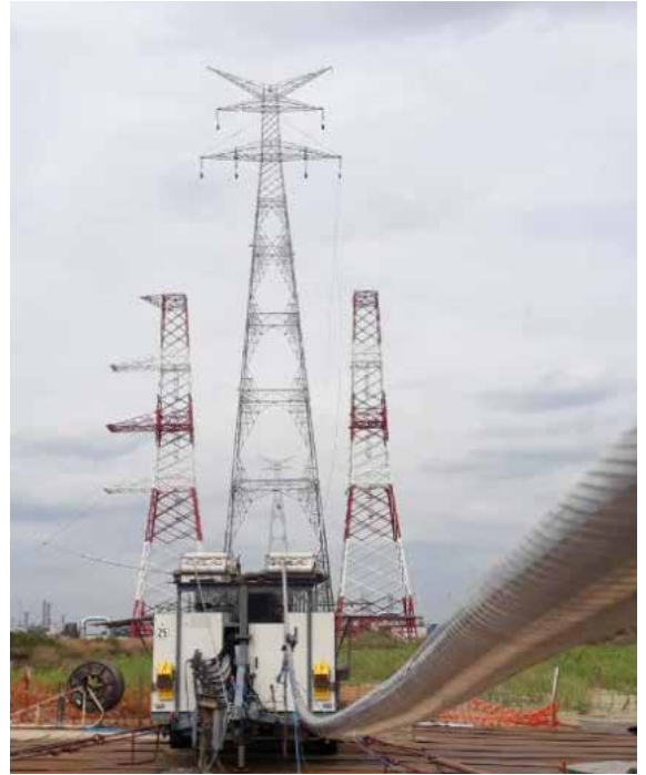
* project data and pictures are used with reference to official CIGRE document B2-203 from 2020
